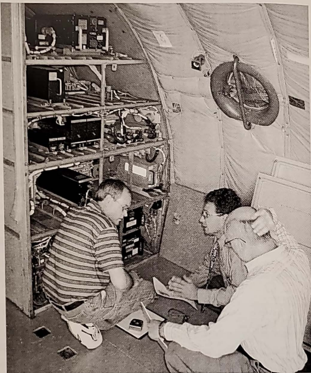
Government contractors take a quick look at the electrical panel in a unit aircraft as part of a fact-finding research effort.
