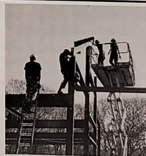
Civil Engineers construct a gymnasium on Indian Territory last May. See story on page 12.
